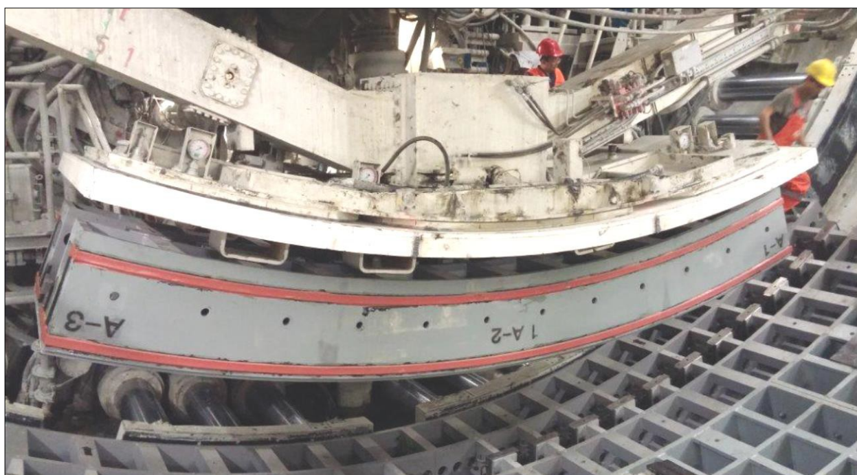
Image 7: Seismic Bracelet Assembly
