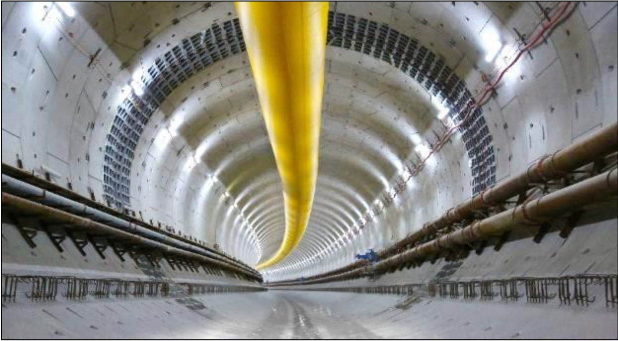
Image 8: Post-Assembly Seismic Bracelets
